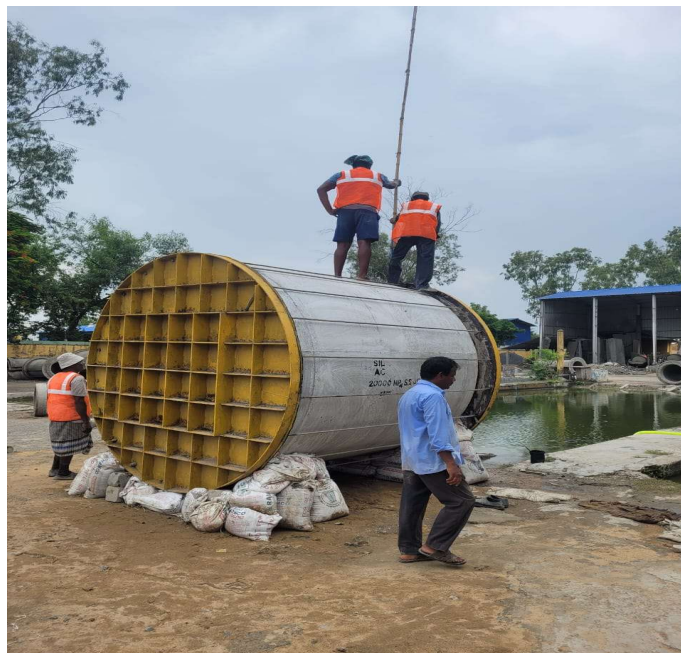
Fig (iv): Hydro Static Test being performed on 2000mm dia NP4 Jack Pushing Pipes
